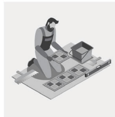
Step-3 Laying of tiles on the Surface
